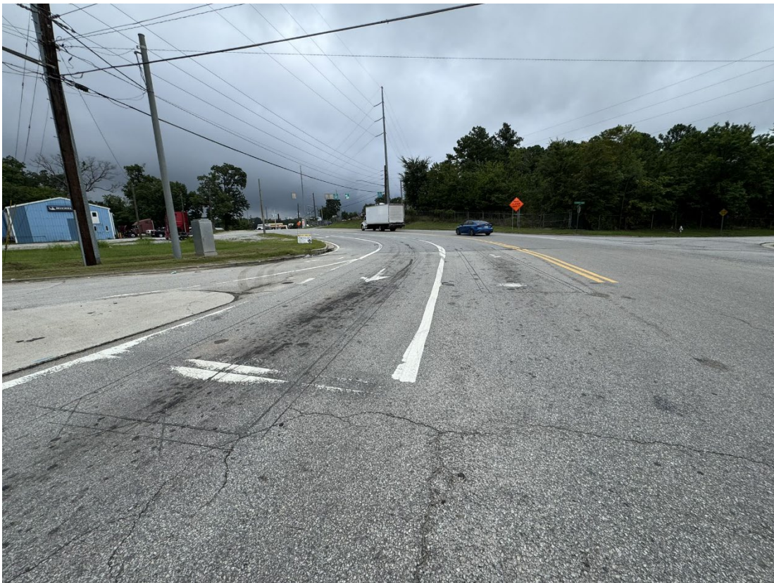
Figure 6: Faded Stop Bar Pavement Markings on East Leg of Intersection (Cedar Grove Rd)
