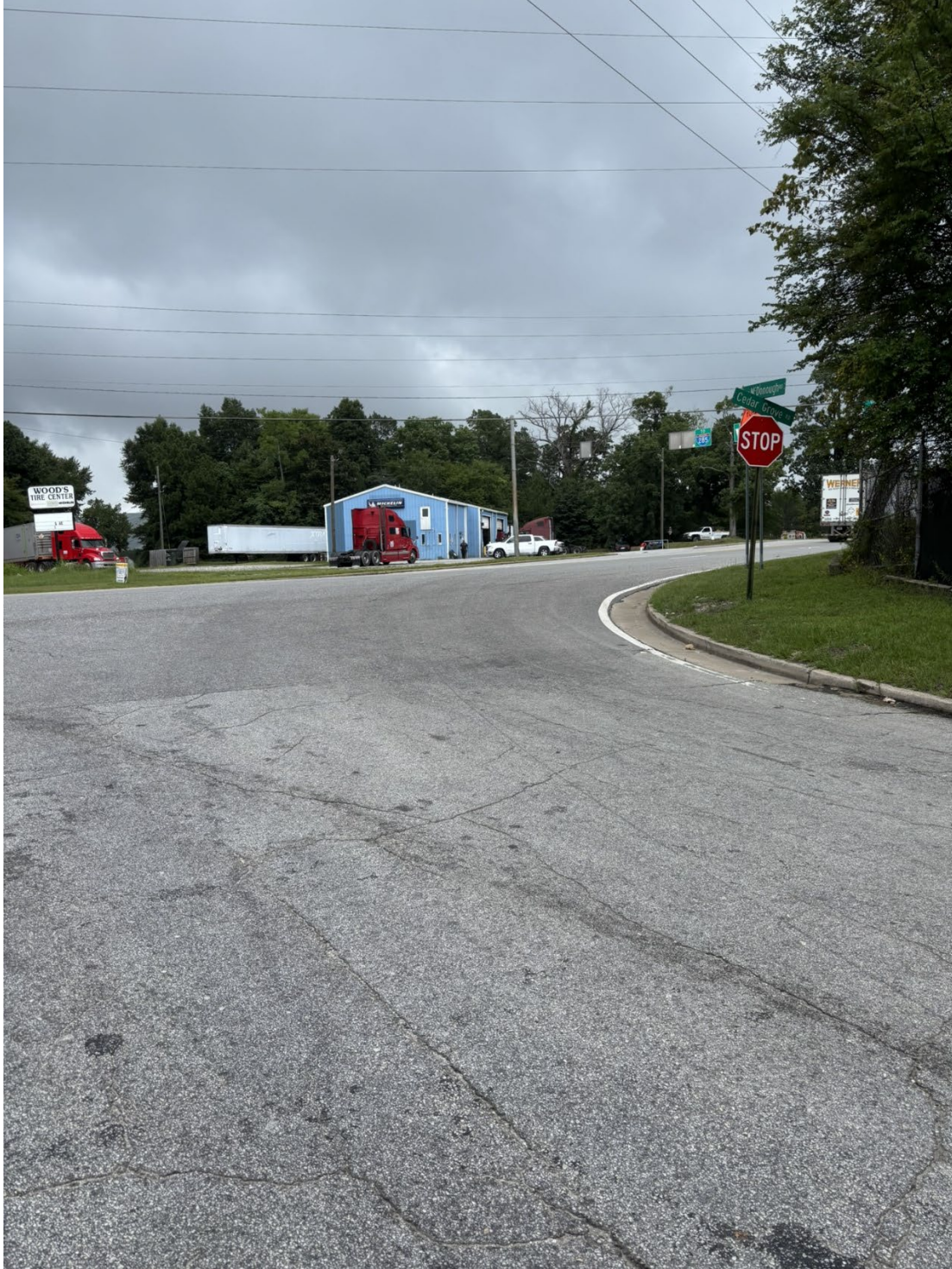
Figure 9: Southeast Intersection Leg Missing Stop Bar (Old McDonough Rd)
