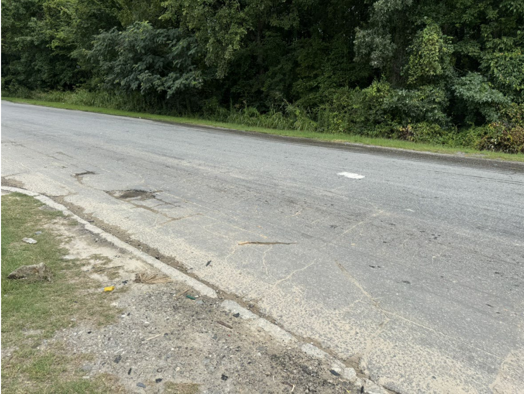
Figure 5: Faded Pavement Marking on West Leg of Intersection (Old McDonough Rd)
