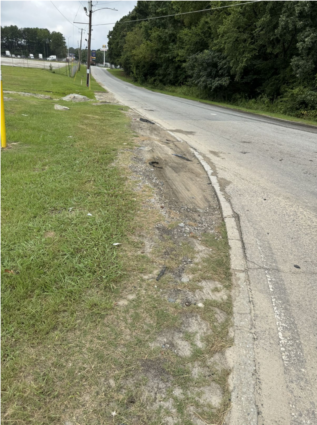
Figure 2: Sunken Curb and Pavement Condition in Southwest Intersection Corner
