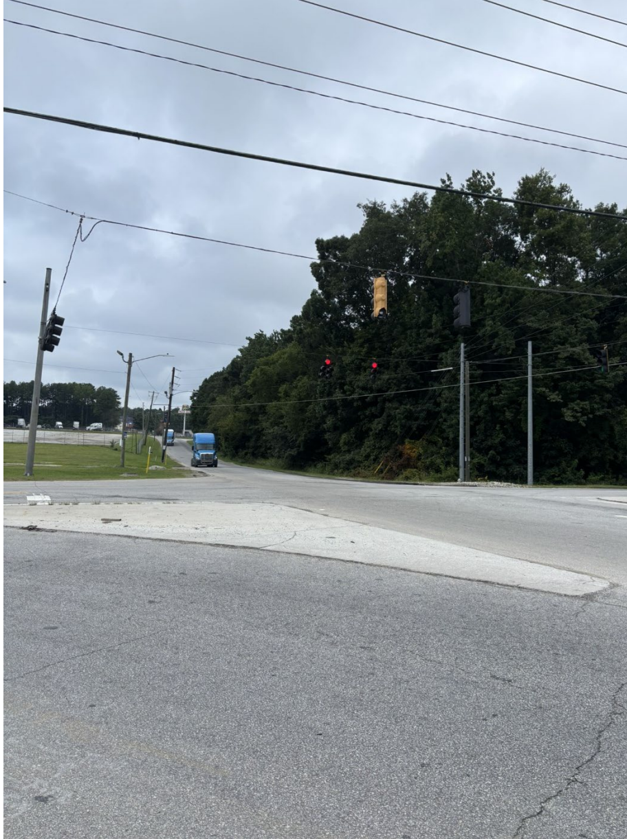
Figure 12: Northbound Channelized Right-Turn Island
