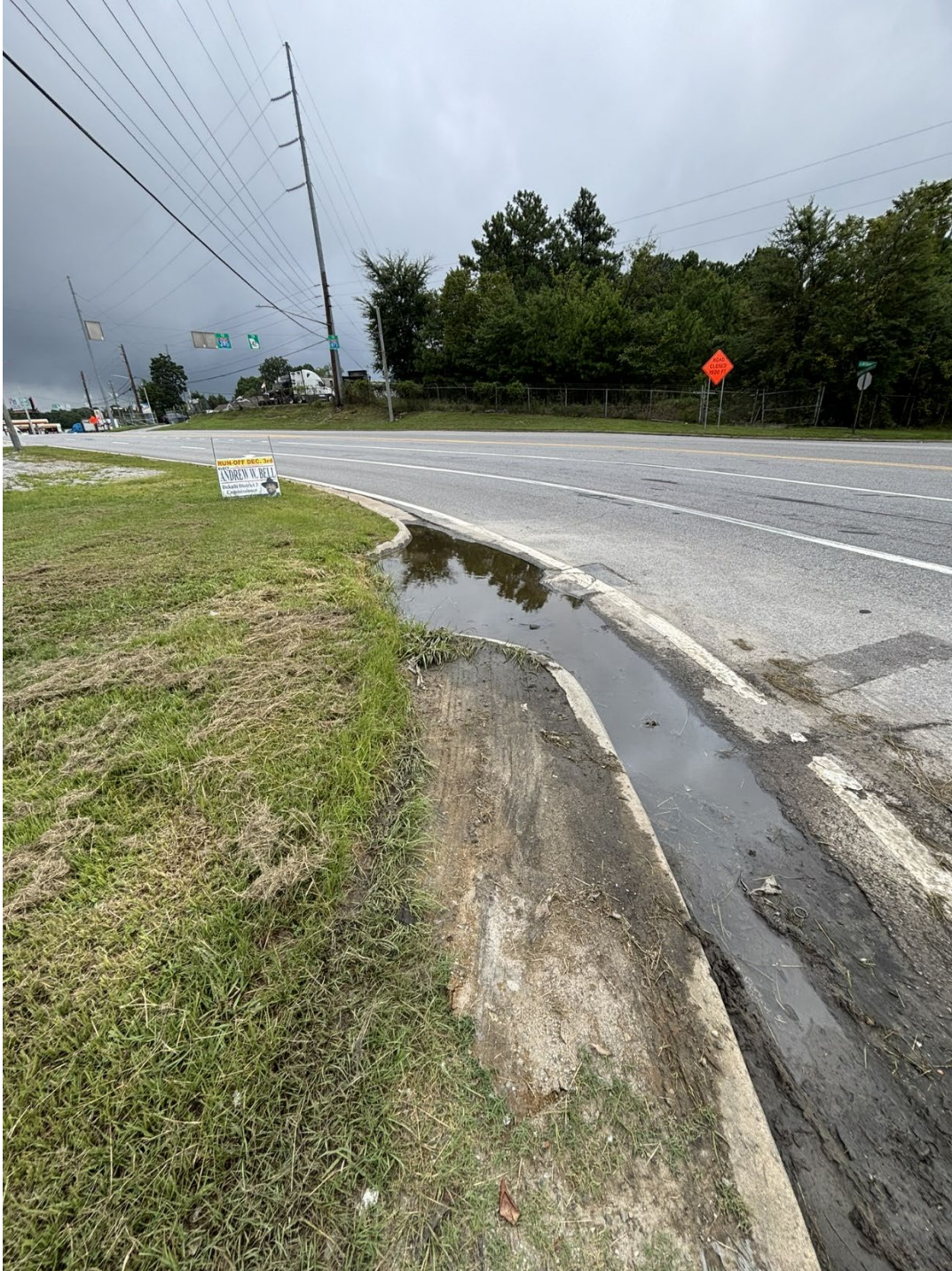
Figure 8: Pooling Water and Poor Drainage in Northeast Intersection Corner
