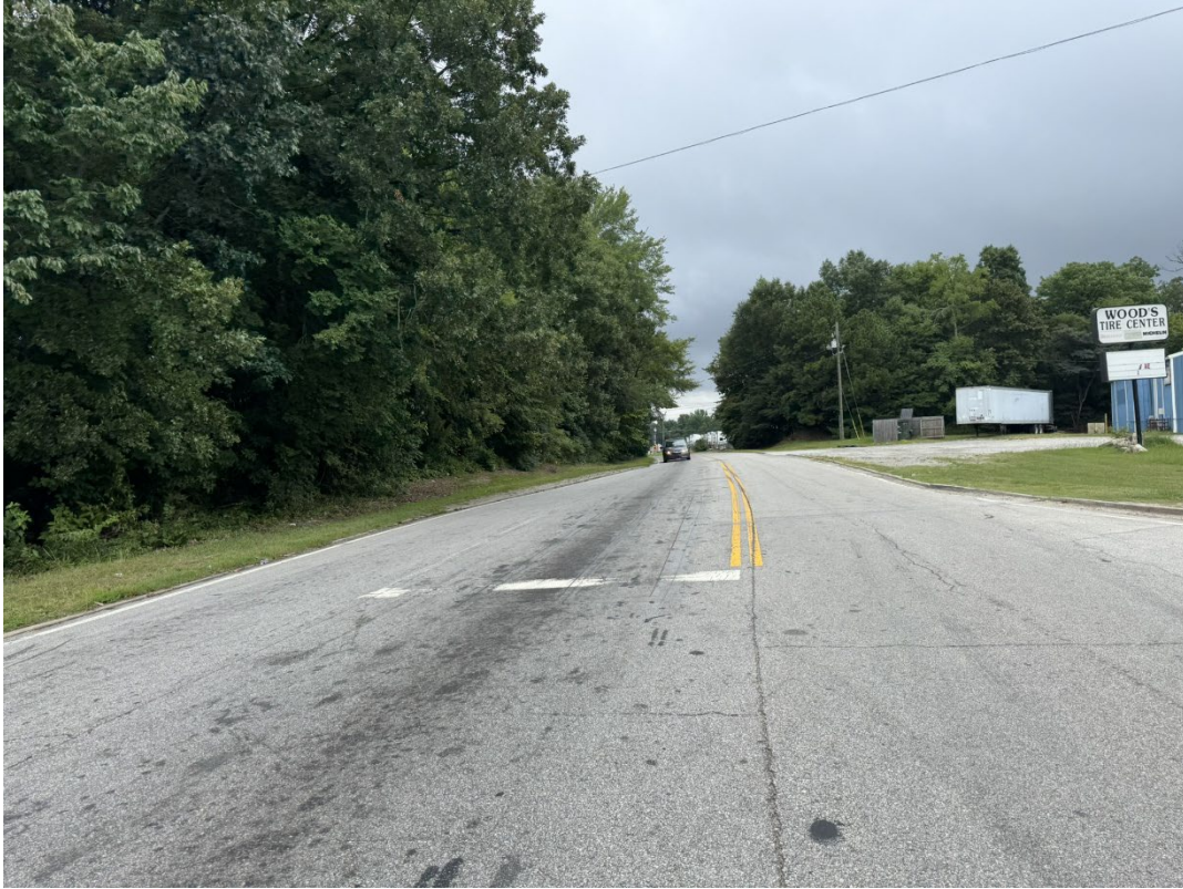
Figure 7: Faded Stop Bar Pavement Markings on North Leg of Intersection (Thurman Rd)
