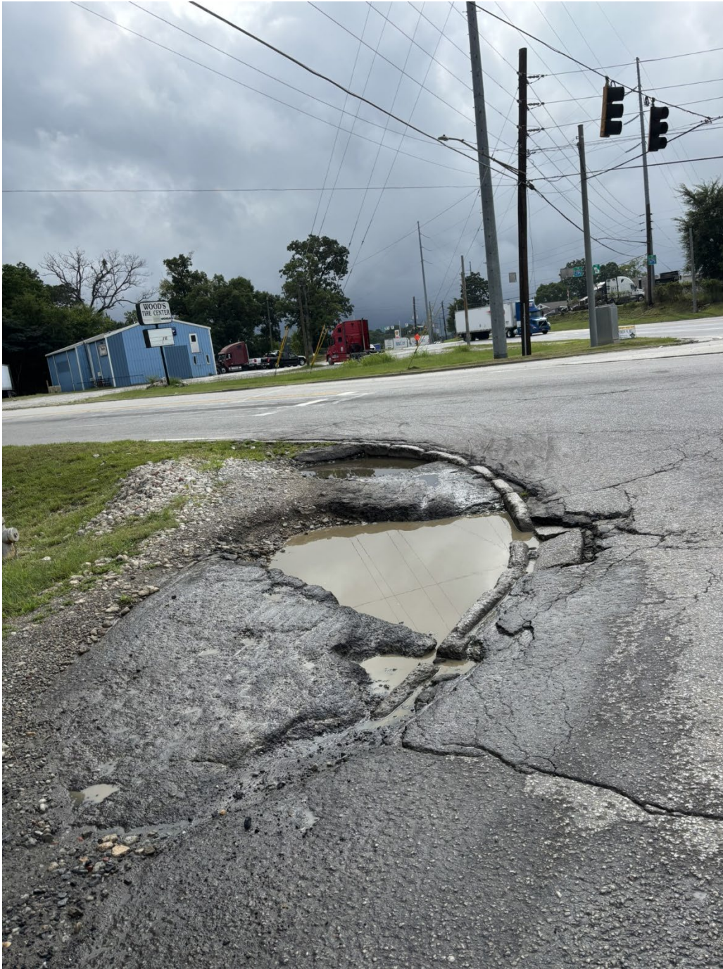
Figure 1: Broken Pavement and Pothole in Northwest Intersection Corner
