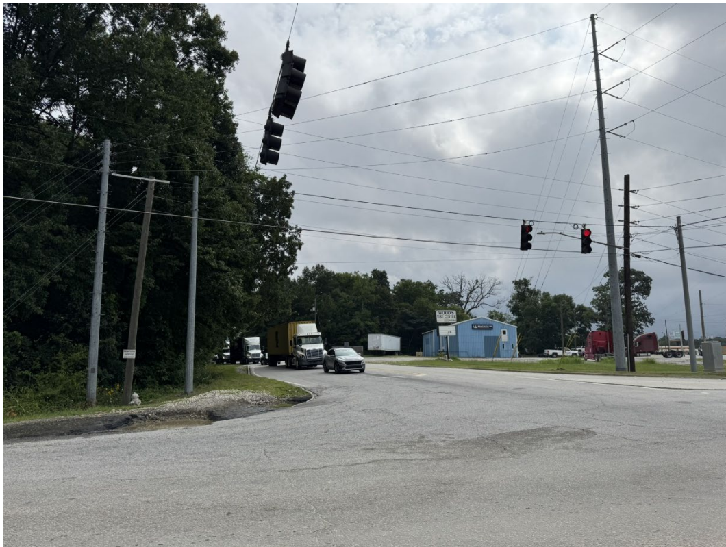
Figure 11: Southbound Outside Lane Underutilization Due to Truck Blockage
